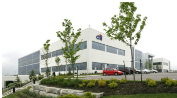
Citi operations centre , Mississauga, Ontario
